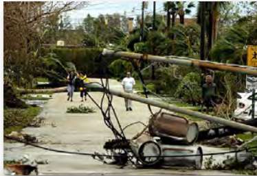
Fallen utility lines after Wilma. From www.galtnile.com
