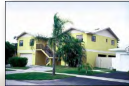
Top Picture: A house in Miami in the process of being elevated. Bottom Picture: That same house once completed. Taken from FEMA, Above the Flood , 2000
