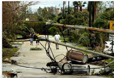
Fallen utility lines after Wilma. From www.galtnile.com
