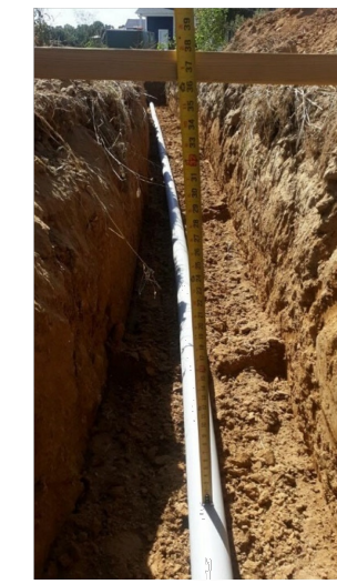
Measurement showing 26" or more cover
