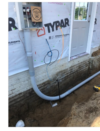
Sweep up into meter pan showing mule tape or pull string
