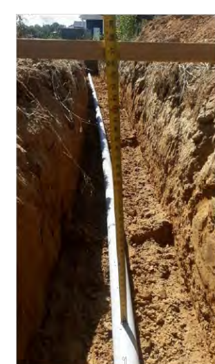
Measurement showing 25" or more cover
