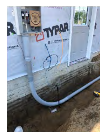
Sweep up into meter pan showing mule tape or pull string
